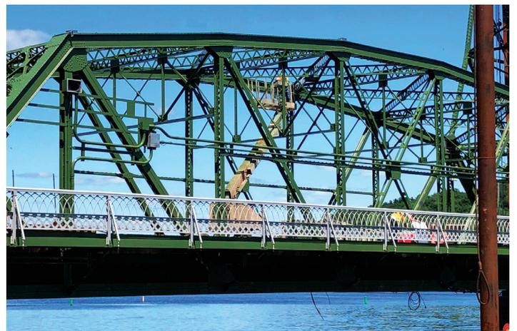
The restoration and conversion of the bridge would include repairing the truss connections, repainting the bridge in its iconic green, rebuilding the concourse, and updating all of the existing mechanical and electrical systems. Mechanical engineers and experts in bridge design were brought in to perform the renovation and ordered over 500 tons of Black Diamond Coal Slag abrasive product to blast through more than a half-century of built-up rust and neglect.
